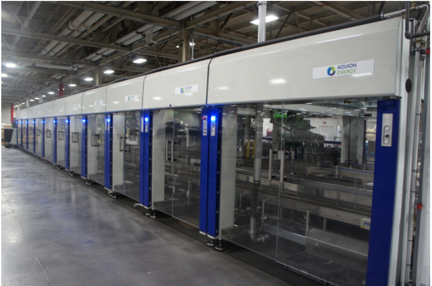
Machines that pick and place the electrodes into the battery units. Image courtesy of Katie Fehrenbacher, Gigaom.
