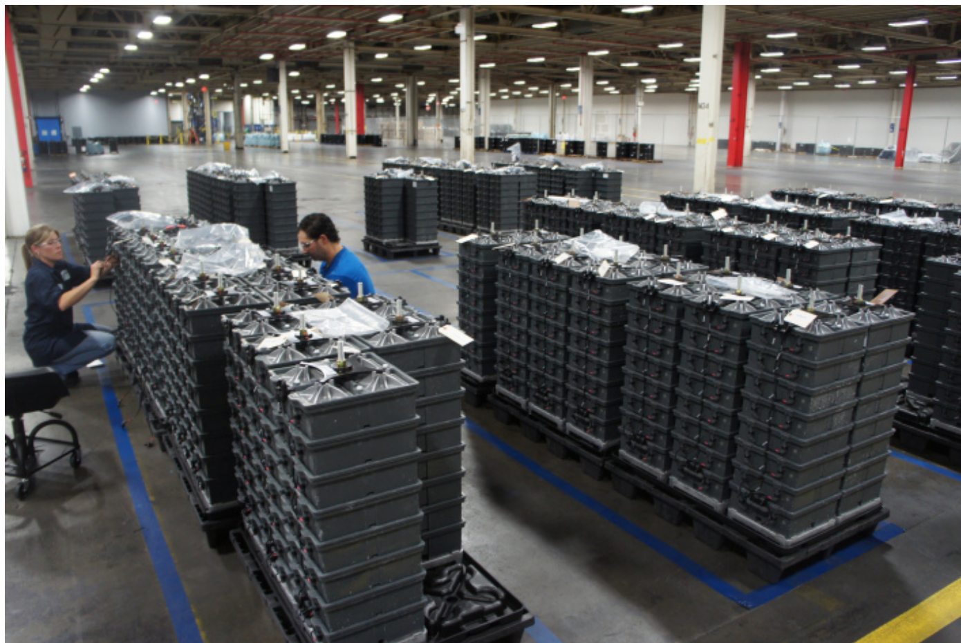
Battery stacks and modules in Aquion Energy's factory. Image courtesy of Katie Fehrenbacher, Gigaom.
